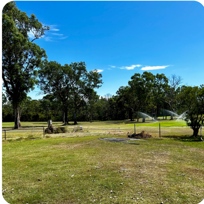
Pictured | Removal of the cricket nets in progress.
